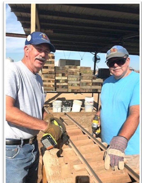
Paul Lator (left) and Joe Fego – Make track panels.
