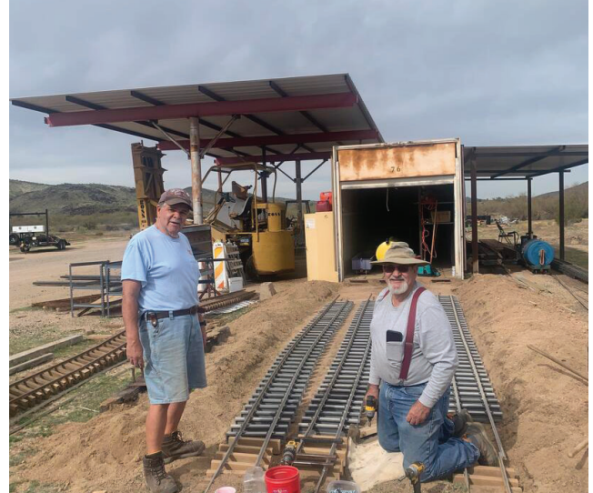
Joe Fego and Craig Danielson laying track into the MoW container.
