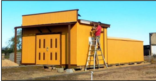
Lewando's Flugel Horn Factory getting some freshening up.
