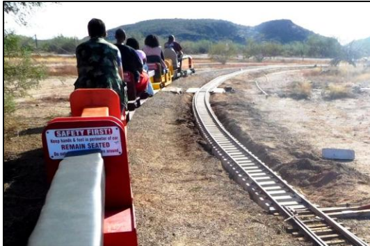
Concrete ties replacing the old, wooden ties at Fisher.
