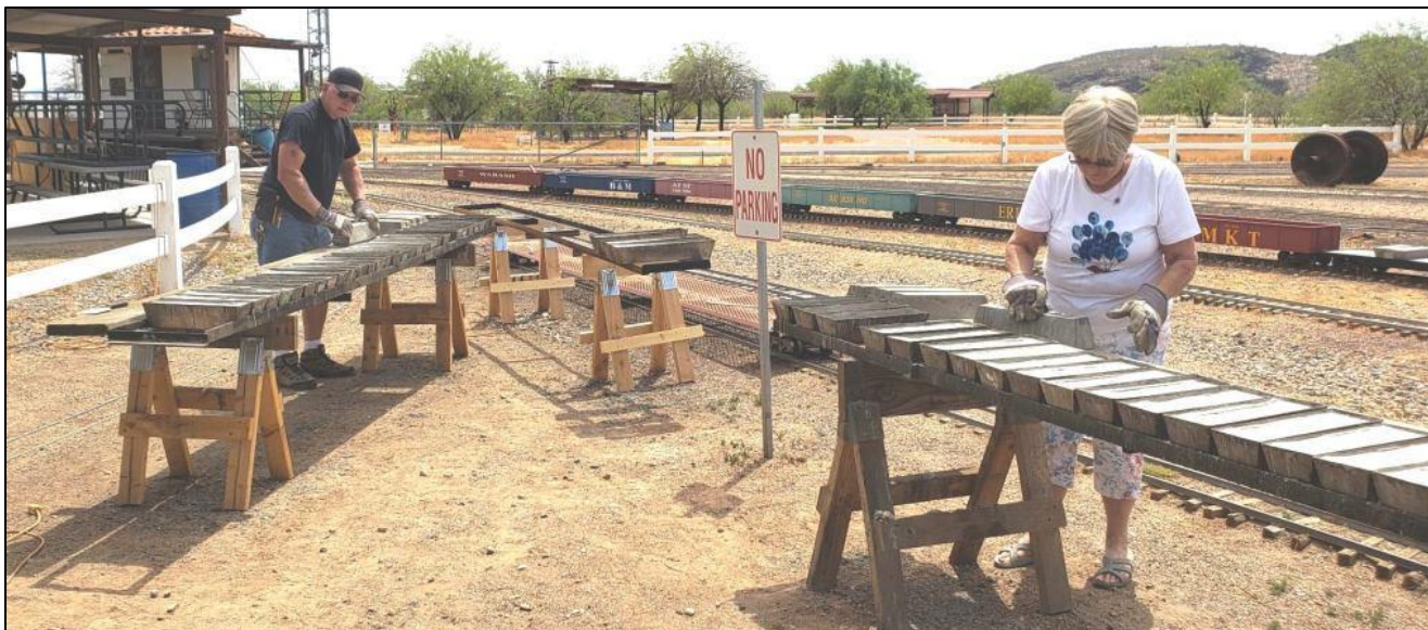
Mike and Judy were making new concrete ties for track repair.
