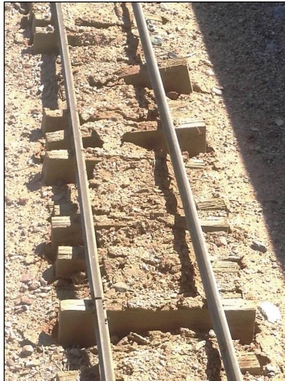
Sunshine under the rails instead of ties
