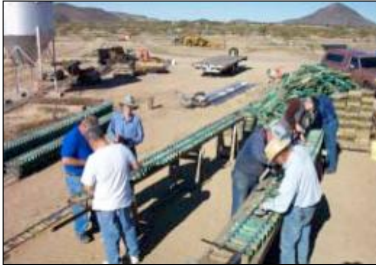
Track Team making track panels.
