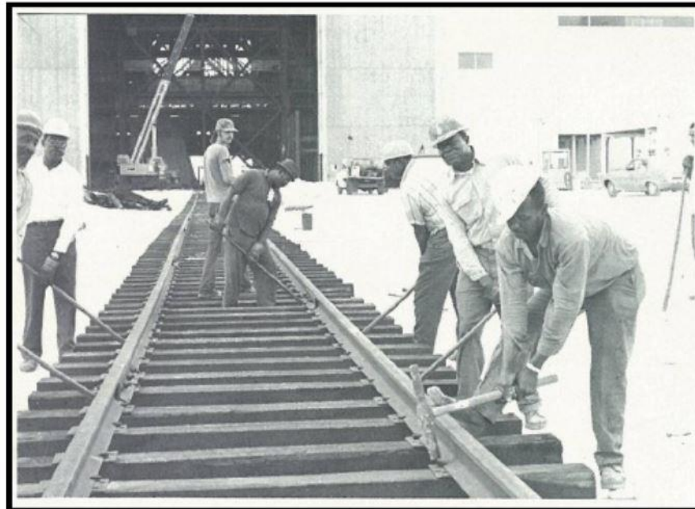
Construction of a spur into the VAB.
