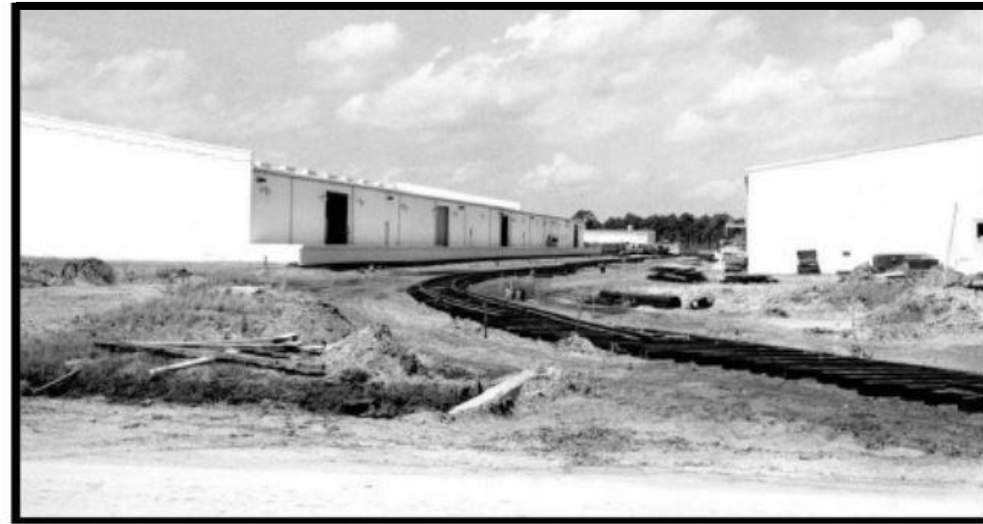
KSC Railroad Construction, 1965. Source: Historical Survey of KSC Railroad
