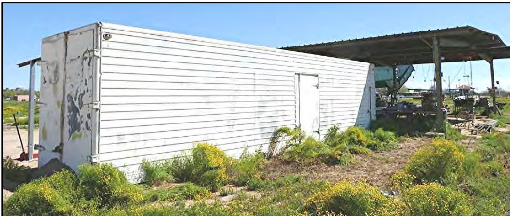
The Sawmill Container (south side) where the supports will be installed for a cover to protect a new turnout storage area, which will be served by a new siding for loading.
