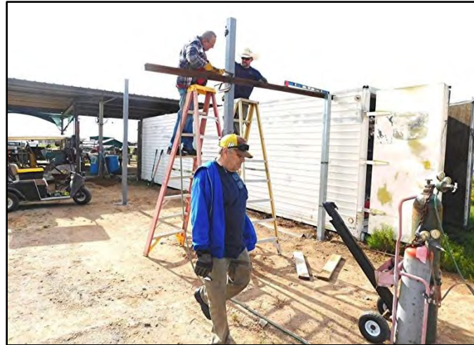
Fred Greenwald, Matthew Rockwell, and Cliff Fought welding the golf cart shed roof cover supports.
