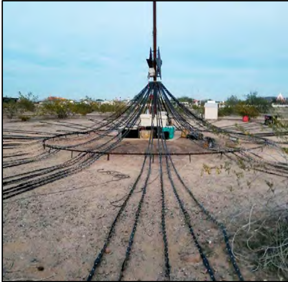
After a short lunch break, it's time to raise the top spindle and connect all 64 light strings to the tree's base ring hooks.
