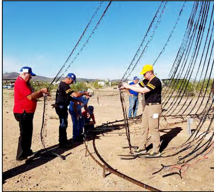
After a short lunch break, it's time to raise the top spindle and connect all 64 light strings to the tree's base ring hooks.
