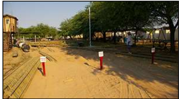
Ready for new panels.
