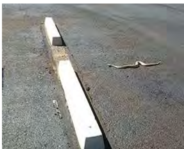
First to cross the new paving!
