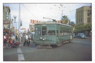
Railway started serving the Phoenix metro in 1887, and at its' peak, went as far as 55th avenue in Glendale from downtown Phoenix. The railway was completely electrified with a line voltage of 550 VDC with, at its' most, 33.8 miles of track and nine lines. To put that in perspective the current Phoenix light rail
